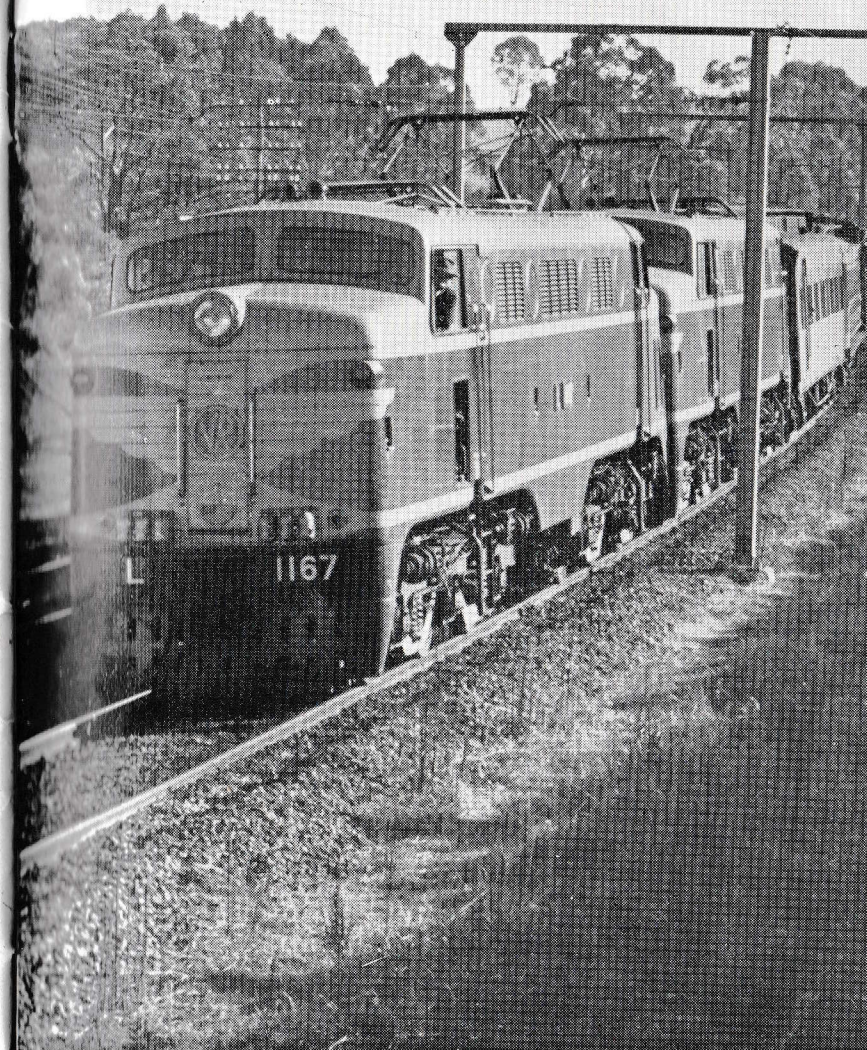
Electric locomotives hauling a test train on the Gippsland line
